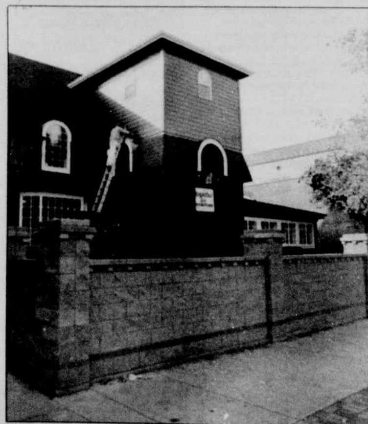
A painter puts the final touches on the newly remodeled Excelsior Inn. Opening in December, the new inn will have 14 new European rooms, each with their own theme.
