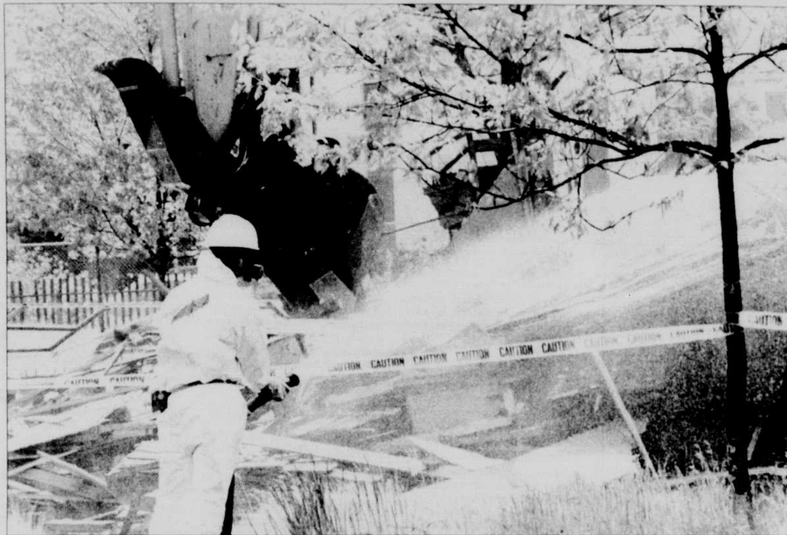
A bulldozer tears down one of three buildings Thursday as contractors worked to clear the site before a stay halted demolition.
