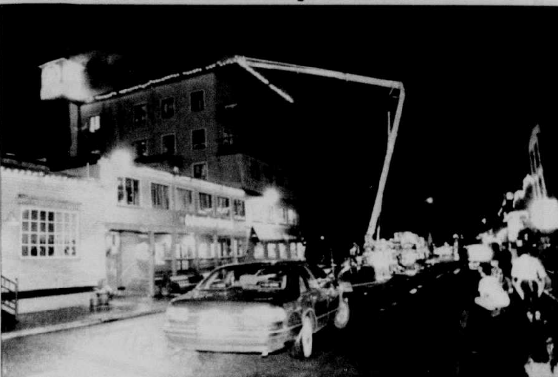
It took fire fighters a little more than an hour to extinguish an electrical fire in the sign tower at the Fifth Street Public Market Friday night. Many merchants said they were not even notified about the fire.
