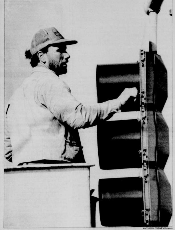
Kevin Ladd of Lantz Electric works on a stoplight at the intersection of Centennial and Mohawk boulevards in Springfield. He added a light for a left turn signal needed for the increased traffic.
