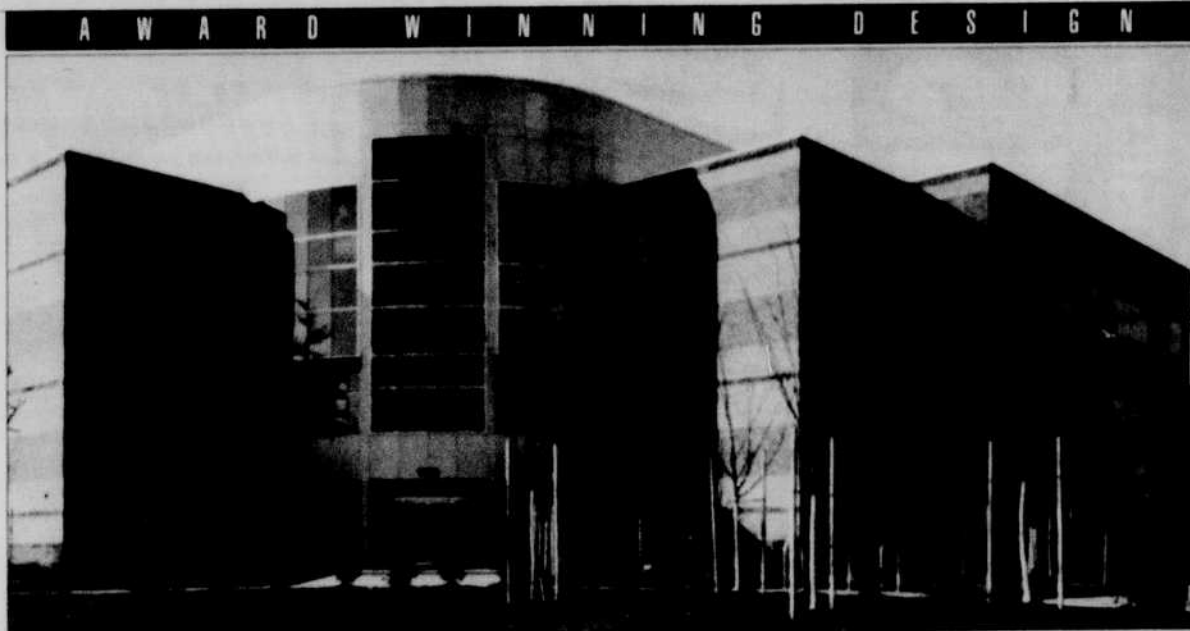
1600 MILLRACE DRIVE RIVERFRONT RESEARCH PARK
