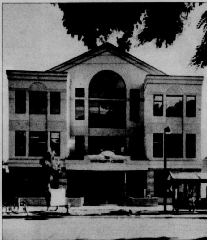
UNIVERSITY CENTER DESIGN STUDIO: BRUCE SINKEY ARCHITECT AIA
