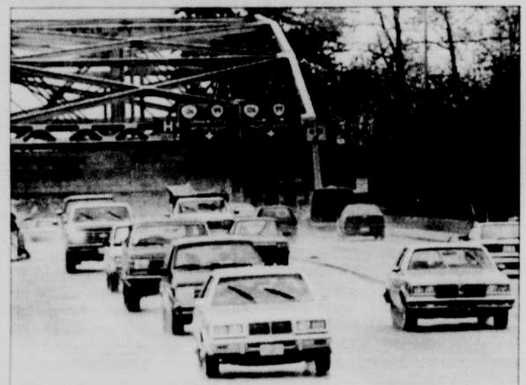
Photo by Jeff Paslay The City of Eugene and a citizen committee have proposed four options to relieve traffic congestion on the Ferry Street Bridge. More than 60,000 vehicles now cross the bridge every day.
