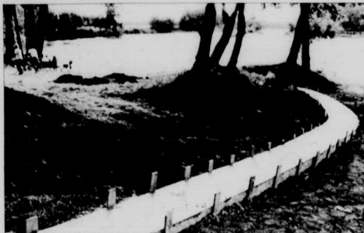
Photo by Brett Matthews
