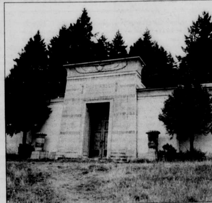
Photo by Derrel Hewitt
