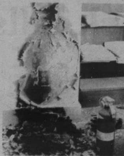
Photo by John Widder At least $500 worth of damage occurred during a fire at Straub Hall last Friday.
