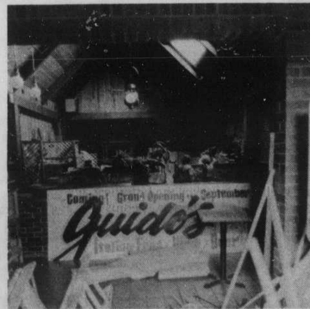
Under construction, the old Duffy's is becoming the new Guido's.
