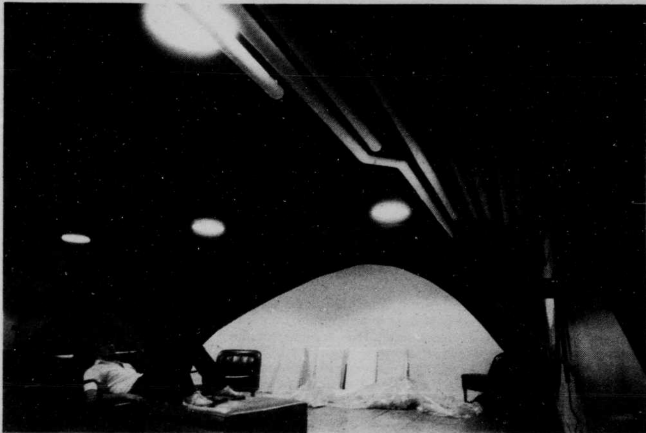
McClure Hall resident Mike Bryce watches TV in the basement of his dormitory. The pipes above his head are insulated with asbestos.
