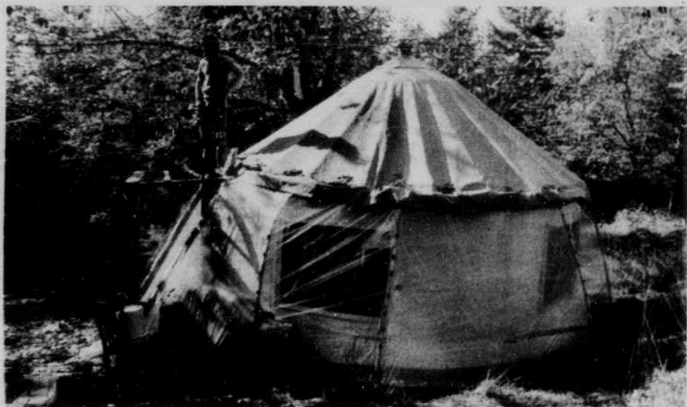
Simone's winterized yurt is covered with a vinyl tarpaulin and wrapped in plastic to protect it from rain and mold.
