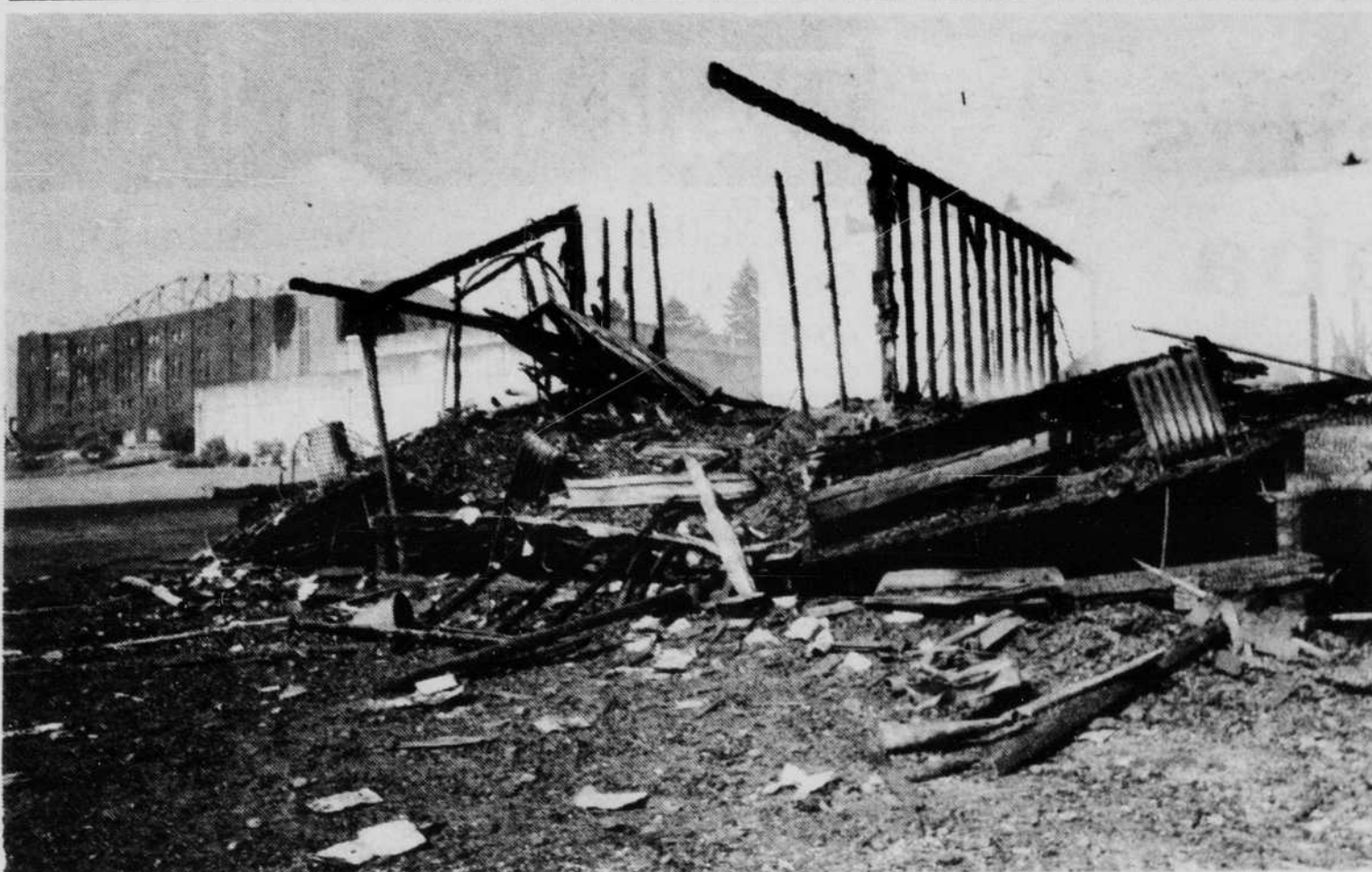
ONCE A SYMBOL of the military's presence on campus, these charred embers of the ROTC building are all that is left after an apparent arson attempt to burn down the office. The attempt, however, was only partially successful, and the Eugene Fire Department burned the remaining skeletal structure. (Archives Photo)
