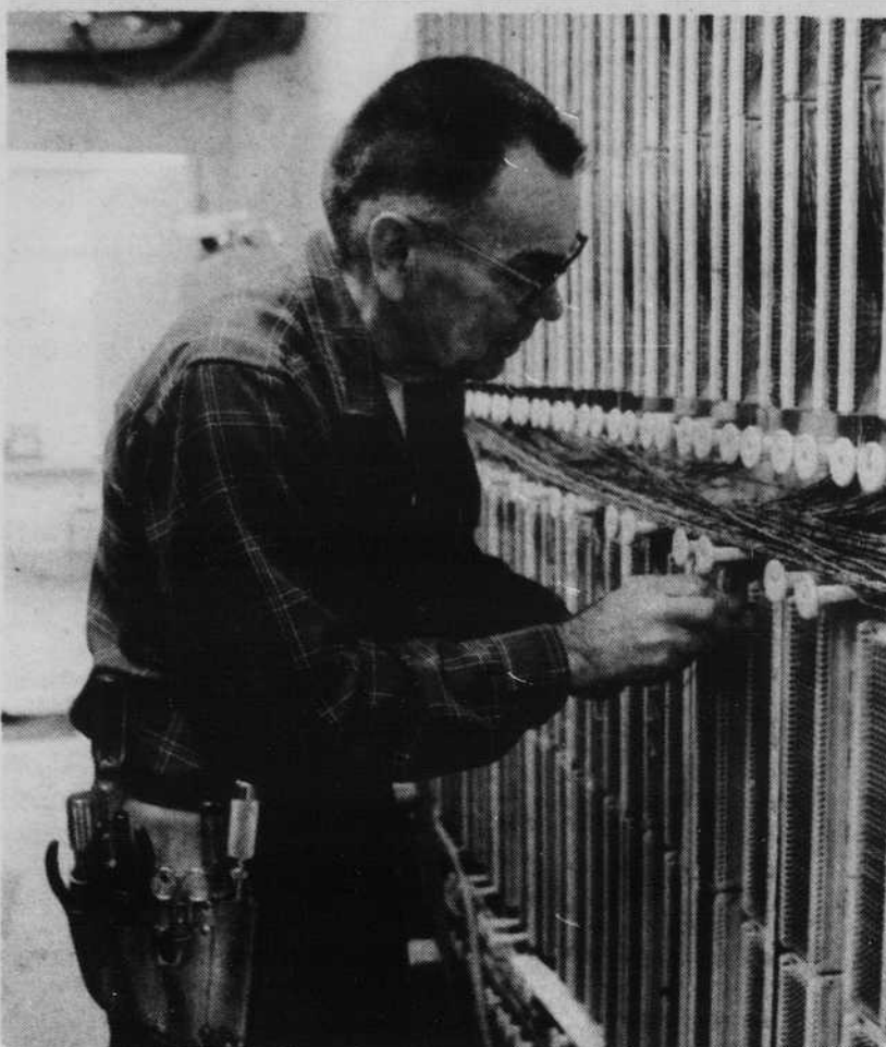
Photo by Trish Weisman Elmer Schultz, an employee of Pacific Northwest Bell, has been wiring circuits in the new Administrative Services Building at the corner of 13th and Agate Streets. The building is occupied, but not yet completed.
