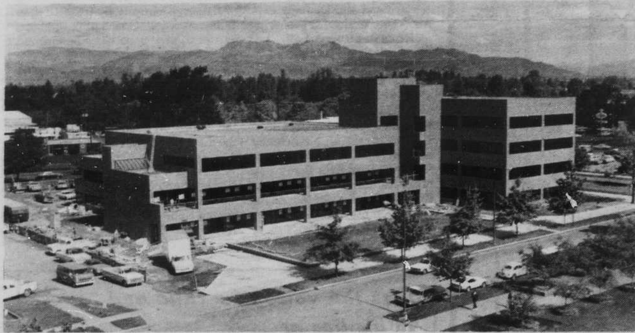
New administration building.
