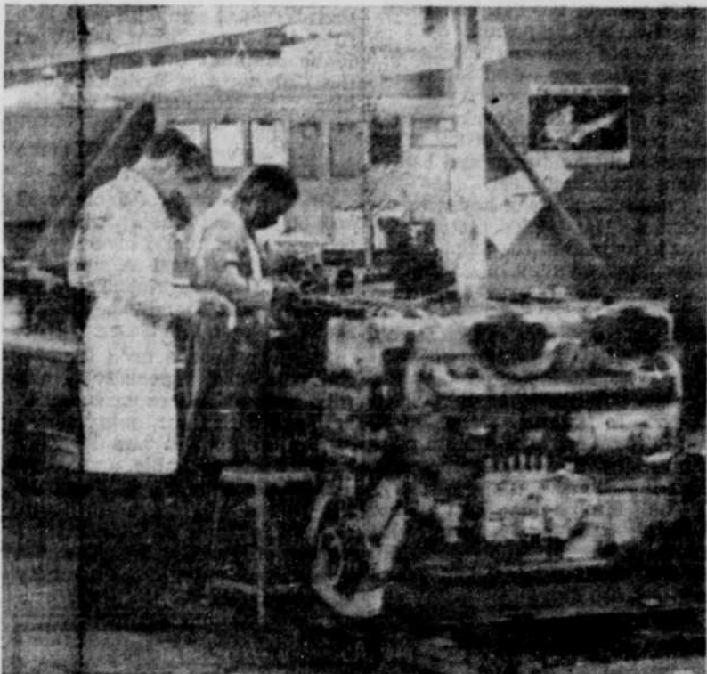
AN INSTRUCTOR (white coat) watches as a Job Corpsman works on an outboard motor in Tongue Point's boat repair division. Instructors attempt to give trainees as much individual attention as possible. The boat motors are used over and over by trainees.
