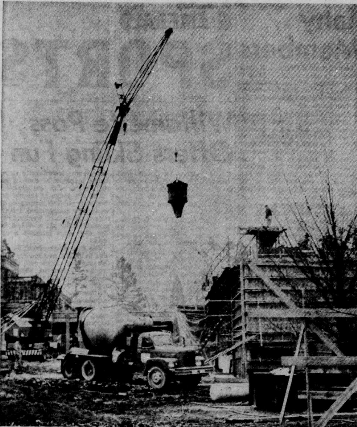
CONSTRUCTION of the new Humanities Building is progressing rapidly, with cement work currently underway. The building is being built on the quad between the University Library and Condon and Chapman Halls.
