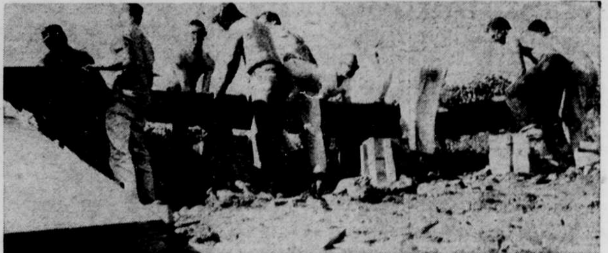
AFTER CARRYING the sections of the "O" down the hill, the task of lining up the edge of the letter with the surveyor's strings proved to be one of the hardest tasks confronted by the work crew. The letter was finally lined up and temporarily bolted together before the final welding of the four connecting joints and remaining legs.
