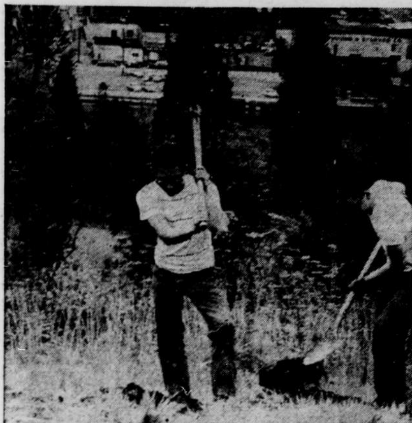
ALPHA PHI OMEGA MEMBERS Francis Fujioka and Jim Hicks work digging holes in bedrock on Skinner's Butte that now holds the piers for the new Oregon "O"—see photo story page 8. (Photo by Louie Parker)
