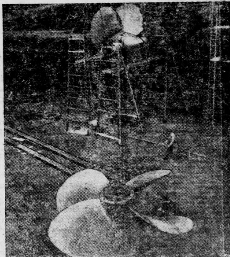
QUEEN'S CHECKUP —Workmen are dwarfed by one of the liner Queen Elizabeth's 32-ton propellers on drydock during annual overhaul of ship at Southampton, England.
