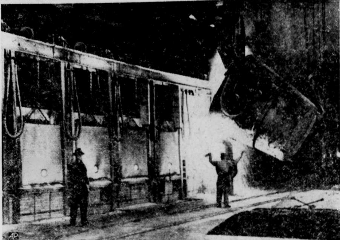
GIANT STEEL MAKER — Molten pig iron is charged into a newly-opened open hearth furnace, the world's largest, at Weirton, W. Va. The furnace is a 600 ton per heat giant.
