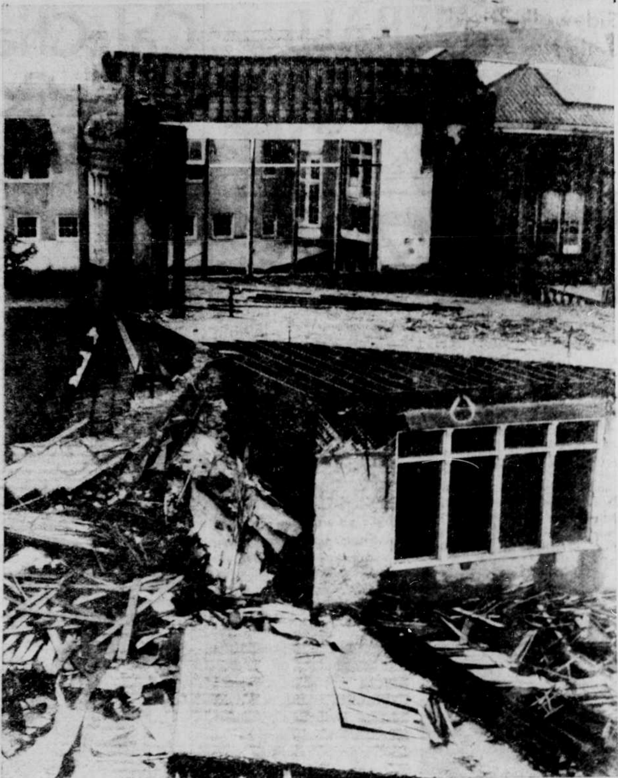
AN' THE WALL CAME TUMBLING DOWN on the old wing of the school of architecture. The building was torn down to make way for a new wing of the school, which is expected to be ready next year.
