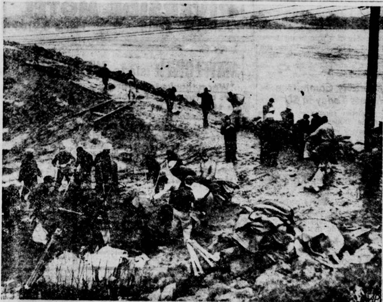
WORKERS FILL SANDBAGS and place them on the bank to strengthen the flood control channel passing through the heart of Long Beach, Calif. Thursday's rainstorm, one of the worst in Southern California history, for a time posed a serious flood hazard to 10,000 homes on the west side of town. At one time water was nearly at the top of temporary levee in foreground. (AP Wirephoto).
