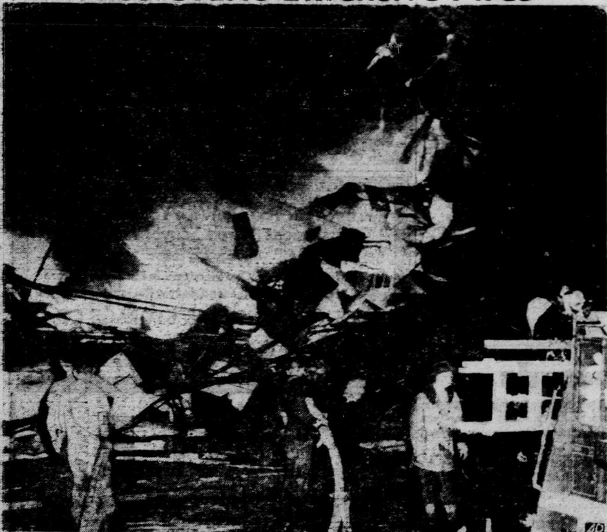
FIRE FOLLOWING A TORNADO destroyed the Hazel Atlas Glass Company plant in Blackwell, Okla., late May 25. The fire and twister combined to destroy the two-block structure as firefighters were handicapped by low water pressure caused by broken water mains. Major Lawrence Youell, a veteran of two wars, said of the ruins in the town, "I've never seen such misery as this." (AP Wirephoto)
