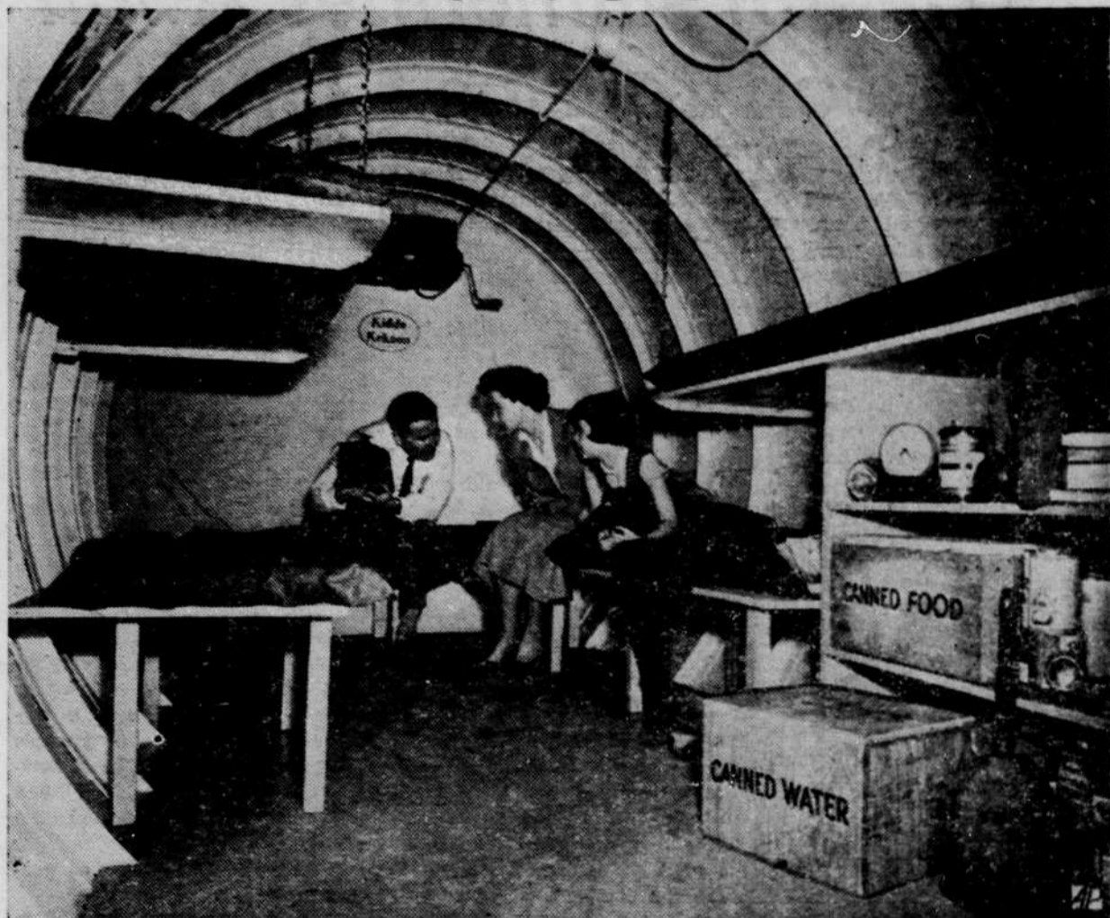
THIS IS INTERIOR of H-bomb steel shelter erected in Garden City, N.Y., whose developers say will take care of a family 3 to 5 days. This deluxe model is equipped with five bunks and air mattresses. At rear of tank is fan which draws purified air through special filter. The handle is used only in event of power failure, which would also necessitate use of battery-powered lanterns. Shelter also has radiation detector, electric battery radio, protective clothing, blankets, crowbar and shovel, first aid equipment plus other apparatus and supplies needed to sustain family. (AP Wirephoto)
