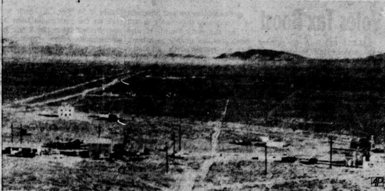
NEVADA DESERT—This picture shows test structures spaced at different distances from ground zero as they awaited the nuclear blast scheduled for today. The first row, including houses and power plant (at right) is 4700 feet from 500-foot tower in which nuclear device is to be set off. Other buildings are at various distances with the big group in background at 10,000 foot position. Pictures were taken with long focal lenses. (AP Wirephoto)
