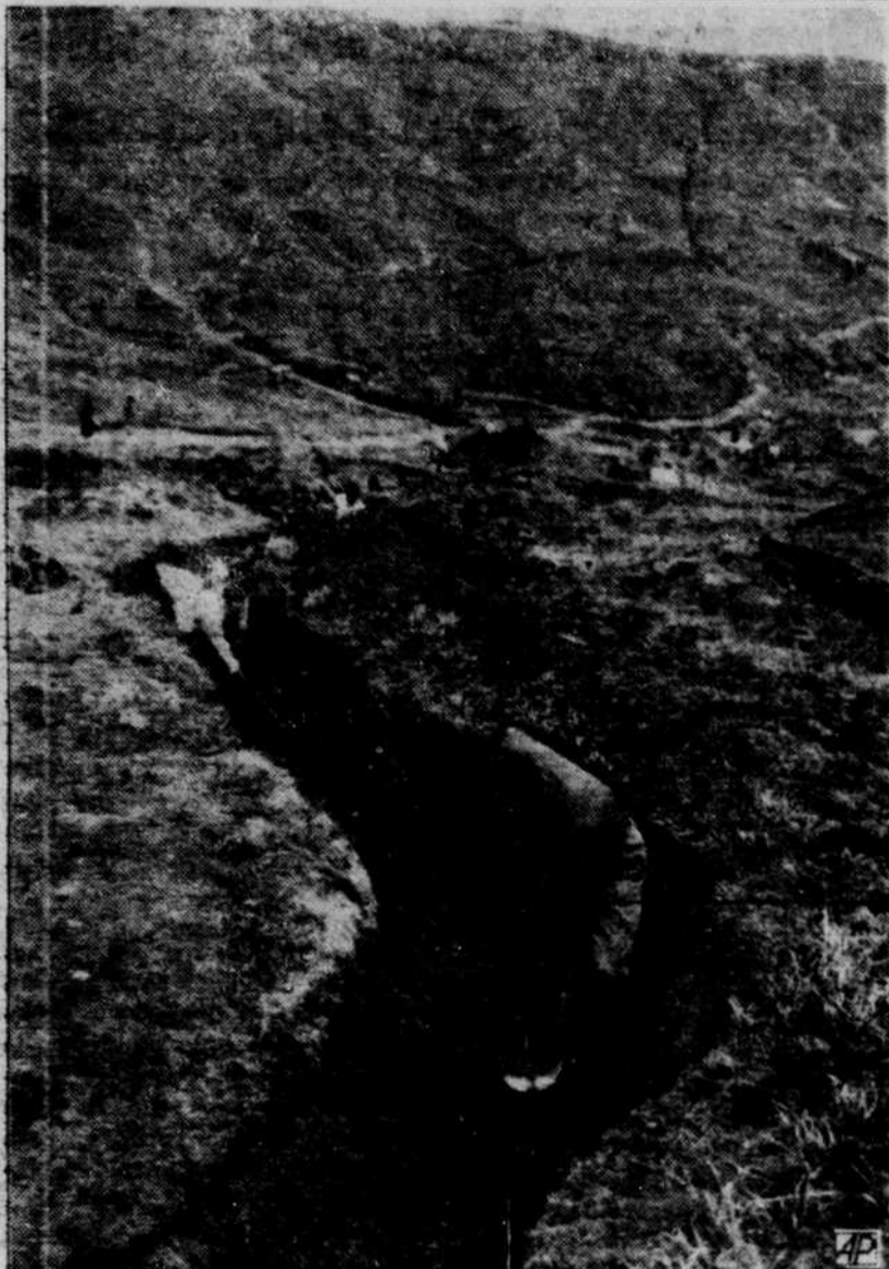
CHINESE NATIONALIST TROOPS dig trenches on Nankan Island, the headquarters island of the Matsu chain. The troops stationed on the islands are building fortifications in expectations of a Communist attack from the mainland nine miles away.—(AP Wirephoto)
