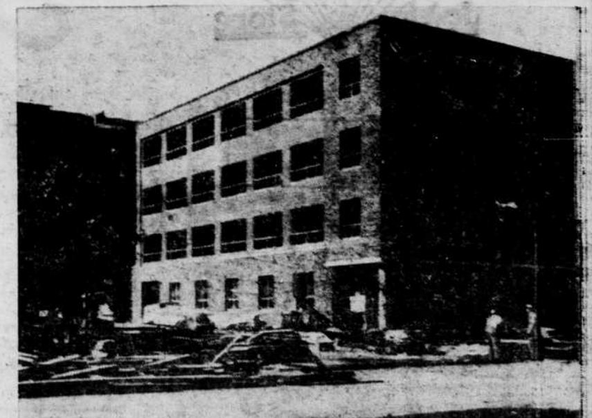
CONSTRUCTION NOISES from Virgil D. Earl hall are familiar to Carson and Straub hall residents. The new men's dormitory was started last spring, and work may be done by fall term, 1955.
