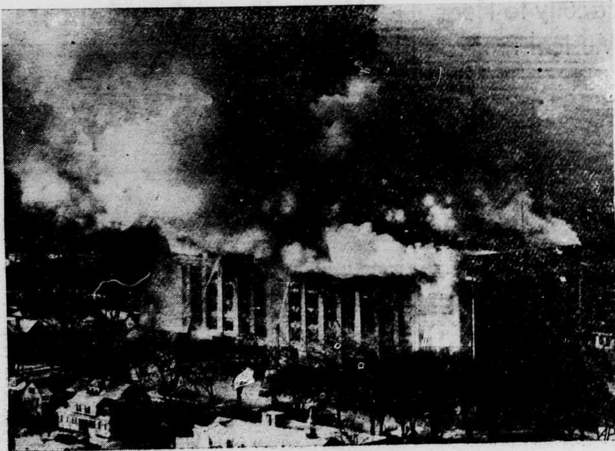
FROM MICHIGAN'S STATE CAPITOL offices smoke billows out in a fire that ragged through the Lansing building for over 24 hours doing an estimated damage of $4,000,000. Below zero weather hampered efforts by five fire departments to fight the blaze which destroyed countless irreplaceable records. (AP WIREPHOTO)
