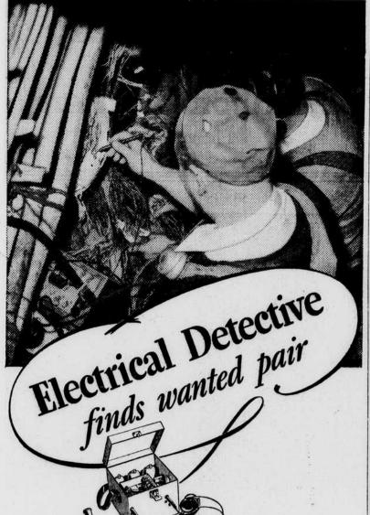
Telephone men know this piece of apparatus as the 108-A Amplifier. It is an "exploring amplifier," developed by Bell System engineers to identify pairs of wires in telephone cables—some of which contain as many as 4242 wires.
