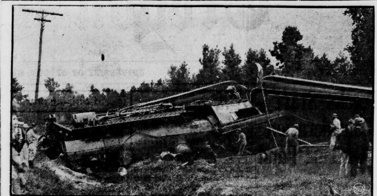
Two men were killed and two were injured in this wreck when the engine and the cars at the head end of a Louisiana and Arkansas Railway train over turned after running through an open switch near Winnfield, La. The railway, beset by a trainmen's strike, was operating trains with outside crews. A student engineer on the locomotive said he saw a man throw the switch when the train was about 400 yards away. Officials of the line said the switch lock had been broken.
