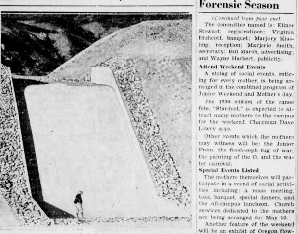
Several wash intakes like the one-pictured will protect the banks ers given by F. R. Sipe, associate of the All-American Canal from flood action-despite the fact that the canal crosses a desert region. The intakes are to take care of cloudbursts. The All-American, to be America's largest irrigation canal, will water large areas in California's Imperial Valley.
