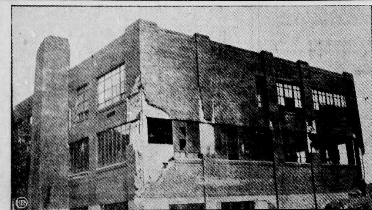
Helena's new half million dollar high school, completed only two months ago, irreparably damaged by a severe earthquake which struck Helena and adjacent territory.
