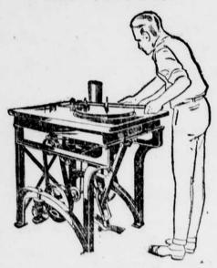
This is called a surfacing machine and is used in grinding the surfaces of either flat or curved rough glass blanks to obtain in the finished lens the exact result required by your individual prescription. This operation requires careful, skilled workmanship.
