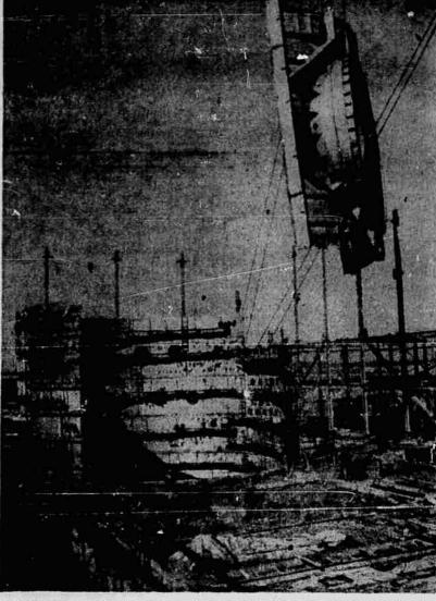
THE 97-TON stainless steel frame (upper right) for the entrance "A" in the Space Environment Simulator Laboratory was lowered into place at the NASA Manned Spacecraft Center's Clear Lake site in Houston, Tex., Friday. The section fits into the open space in the chamber at lower left. (UPI Telephoto)
