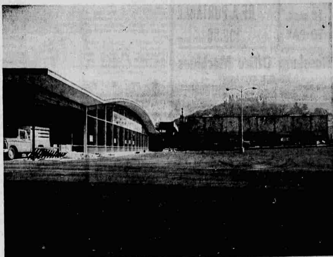
PLAZA GOES UP — One of the most satisfying sights to a lot of Roseburg people this year was the construction being carried on in the heart of the city on a new shopping center, Roseburg Plaza. Here in a late stage of construction looking across the big
