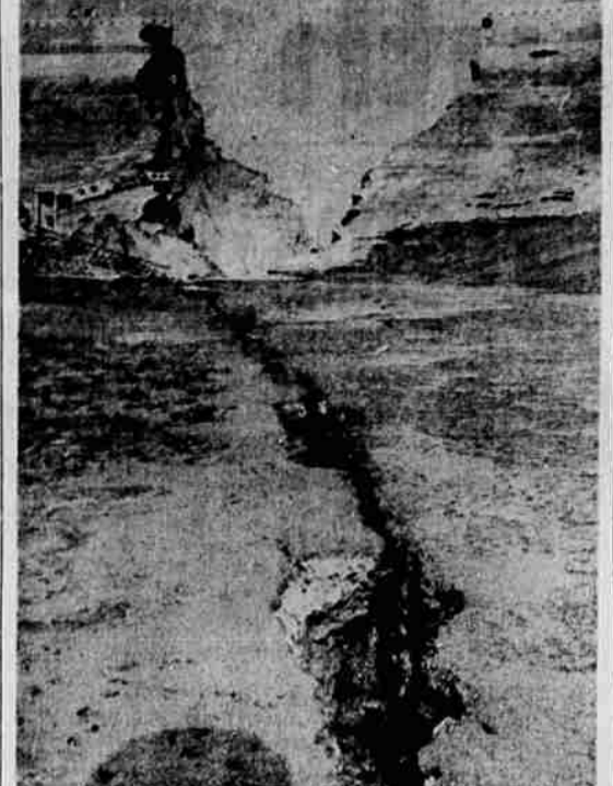
THIS HUGE CRACK , discovered at the bottom of the Baldwin Hills Reservoir in Los Angeles, is believed to be the basic cause of the collapse of the dam and its subsequent destructive torrent of water that left three dead and property damage over the $10 million mark. (UPI Telephoto)
