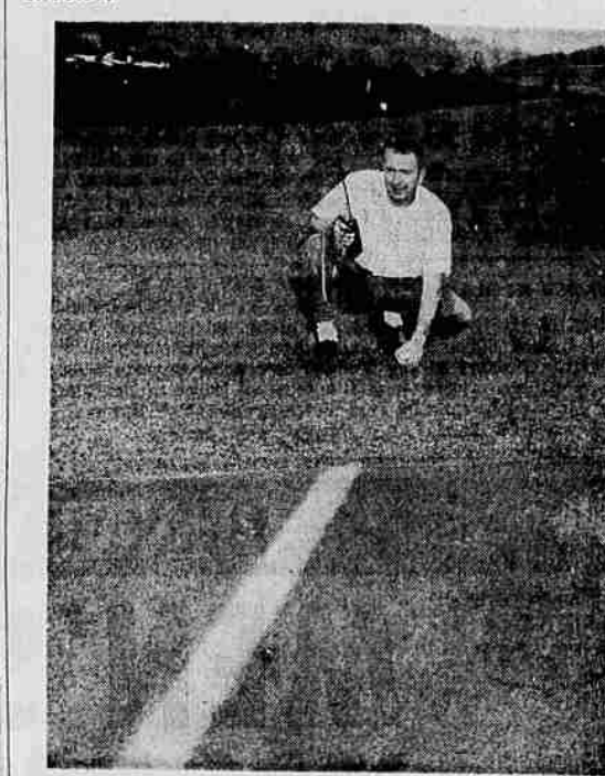
RE-STRIPING airport runway and taxiways was required following surfacing improvements. Above Don Staebler, assistant city engineer, marks newly surfaced area to be striped after center line location is determined by instrument reading. Reflectorized center line for runway and taxiway is required by Federal Aviation Agency.
