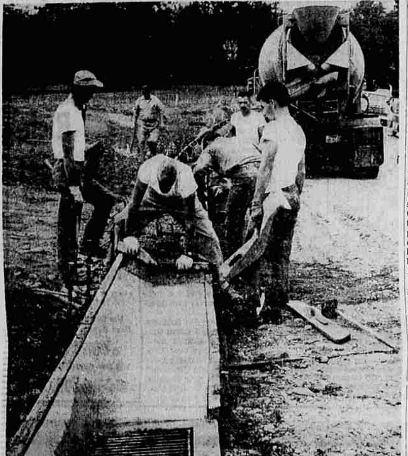
CREW OF FRED STUBBERT, subcontractor to Roseburg Paving Co., is shown pouring curb structure for the new West Oriole-Bradford street paving improvement. City officials said the subcontractor last week was pouring 1,200 feet of curb per day. The contractors are racing against the weather to get the project completed.
