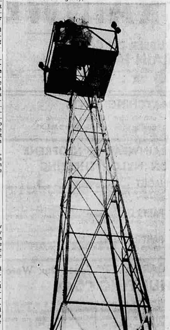
BOB SCOTT is shown in a lofty position as he replaces burned out bulb in beacon light at Roseburg Airport. Maintaining these lights is one of the Public Works Department's many responsibilities. Cost of a beacon bulb is $14.
