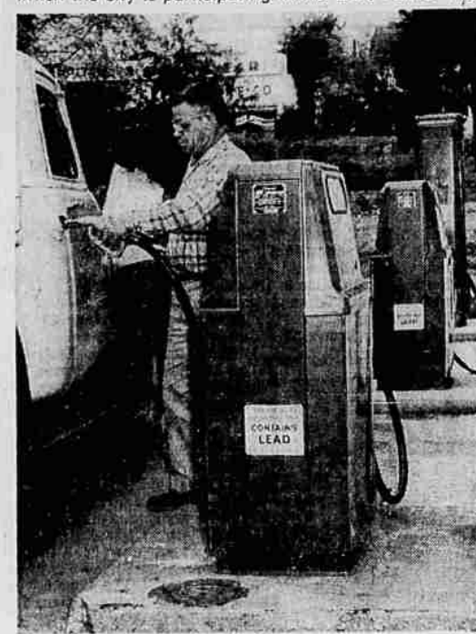
GEORGE SCOTT, superintendent at the city shops for the past eight years, fills pickup with gas from newly installed pump at the shop yards. New ethyl and diesel tanks and pumps were installed at the facility this year.
