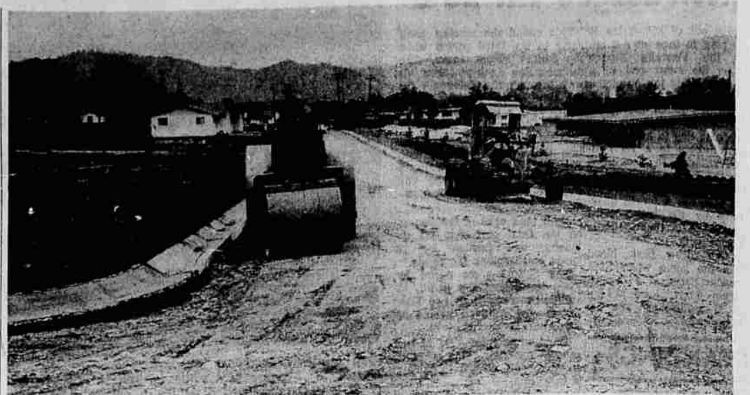
MEN AND EQUIPMENT of Roseburg Paving Co. are shown at work on West Bradford Drive where a street improvement is in progress. The Bradford-Oriole project is an assessment district activity in which the city is participating in the cost. Part of the
