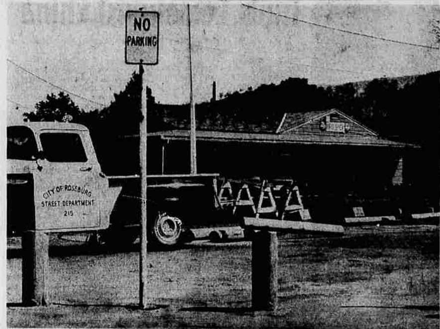
GUARD POSTS have been installed at both ends of the street segment in front of the Stewart Park pro shop in connection with the establishment of a parking area in that street and the re-routing of Stewart Park Road traffic around the Pavilion loop. A couple of the guard posts can be seen above. In background can be seen logs which are being used in the preparation of 11 new parking stalls. The "No Parking" sign is in reference to the area near the guard posts just outside of the parking zone. (News-Review photo)
