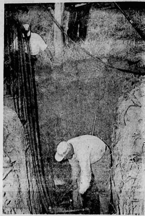
DRILLING RIG — Clyde Marriott, Glendale business man, and his father, Ivan Marriott, retired, Sacramento, Calif., and Glendale, are shown with drilling equipment working in a ditch where he bored 90 feet under the highway in six hours. Marriott senior is shown removing pipe sections connected to the hydraulic pumping plant on the ground level. (Fox Studio)
