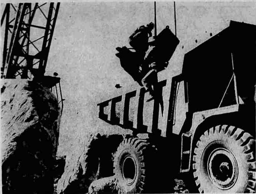
BIG is the word for all impressions about the modern Umpqua South Jetty building operations. Big rocks, big equipment, big men and big motions do the big channel-directing work of the jetty. Here tongs, broken on big rocks of 19 to 40 tons, are changed.
