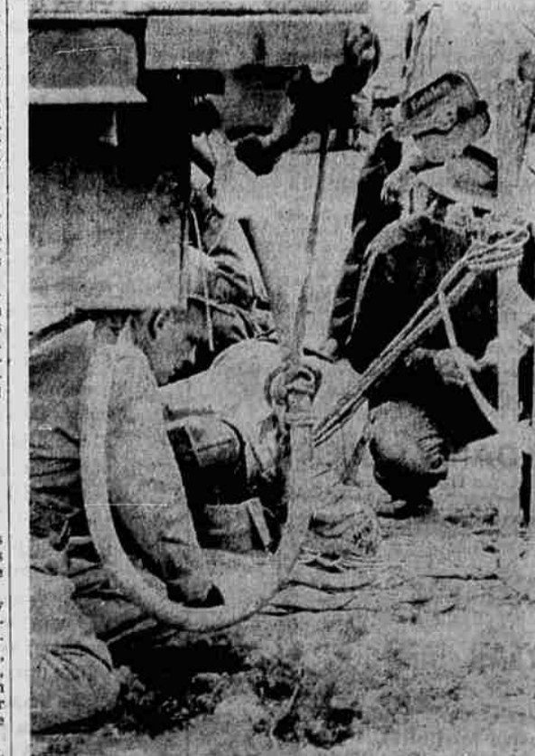
RESCUE WORKER presses his ear to the six-inch pipe through which communication and supplies are maintained with trapped miners in Pennsylvania coal mine, some 300 feet below the surface. Two of the trapped miners communicated with the third in another part of the shaft, by tapping on the wall and told rescuers the third man was injured, but not covered with rock. (UPI Telephoto)
