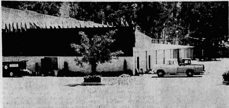
ADDITION COMPLETE — Work has been completed in time for the Douglas County Fair on the addition to the Livestock Pavilion at the Fairgrounds. The addition gives 4,000 more square feet for pens for livestock exhibits. During the off-season, it will be used for storage. Also included in the addition are restroom facilities which double the number available at the Fairgrounds before. (News-Review photo)
