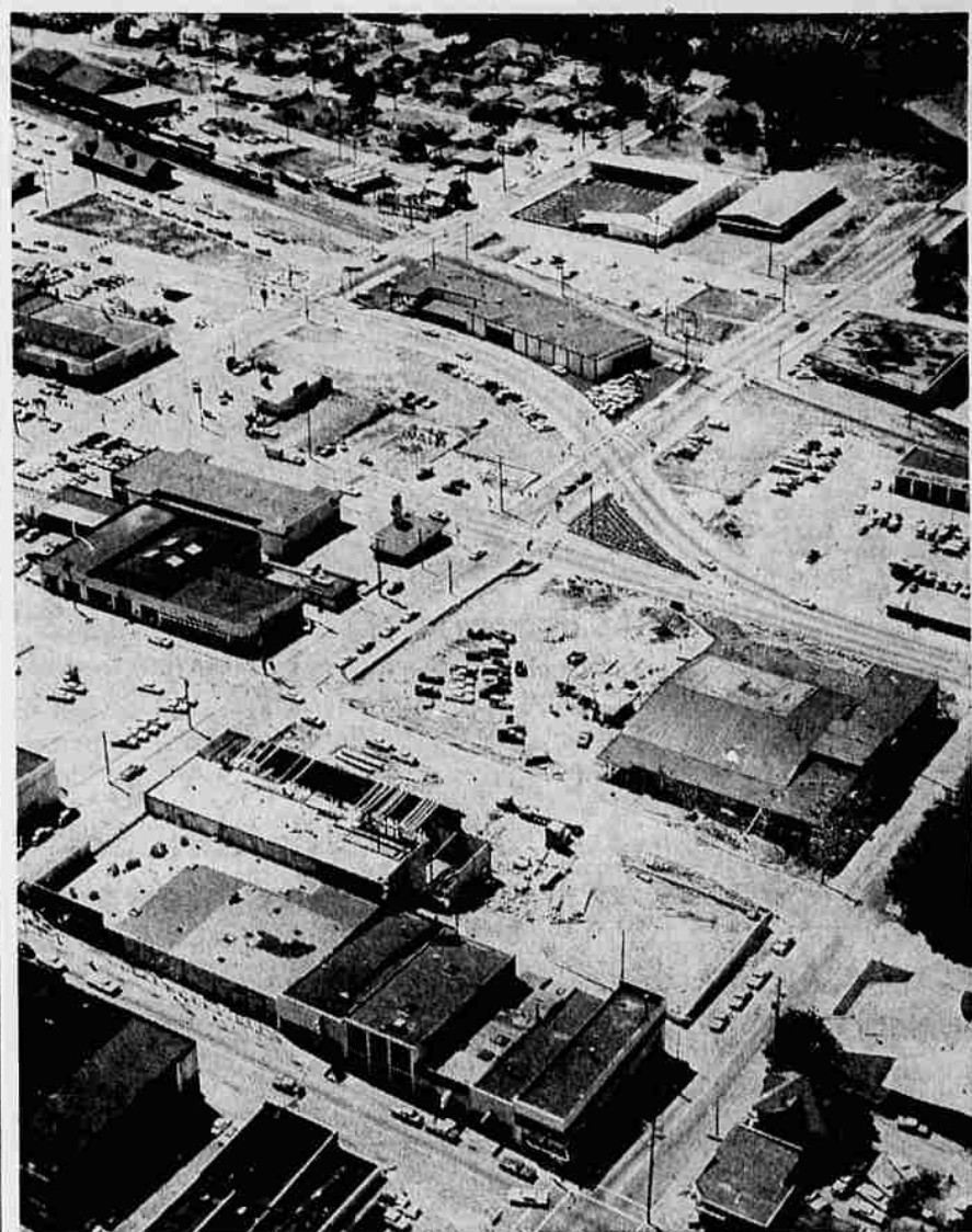
BLAST AREA REBUILT — Four years after the blast which tore out a big section of the city, a transformation has taken place. The aerial photo by News-Review photographer Andy Fautheree was taken from a helicopter. Cutting through the center of the area is the new SE Pine-Stephens couplet. The U-shaped building at upper right center is the new Holiday Motel, flanked by the Farm Bureau warehouse. The long building just below it is the new Lockwood Motors Co. structure just opened for business. The Central Junior High School property is now being changed by the construction of Roseburg Plaza. It includes a new Safeway store (right center, below the merging point of Pine and Stephens) and a new Pay Less store, lower left.
