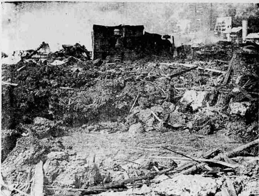
THIS YAWNING CHASM , 20 feet deep and 50 feet across, marks the parking place of the Pacific Powder Co. truck which exploded here Aug. 7, 1959. This is the site of Lockwood Motors new building, the crater being about midway of the property. A marker is to be placed there.
