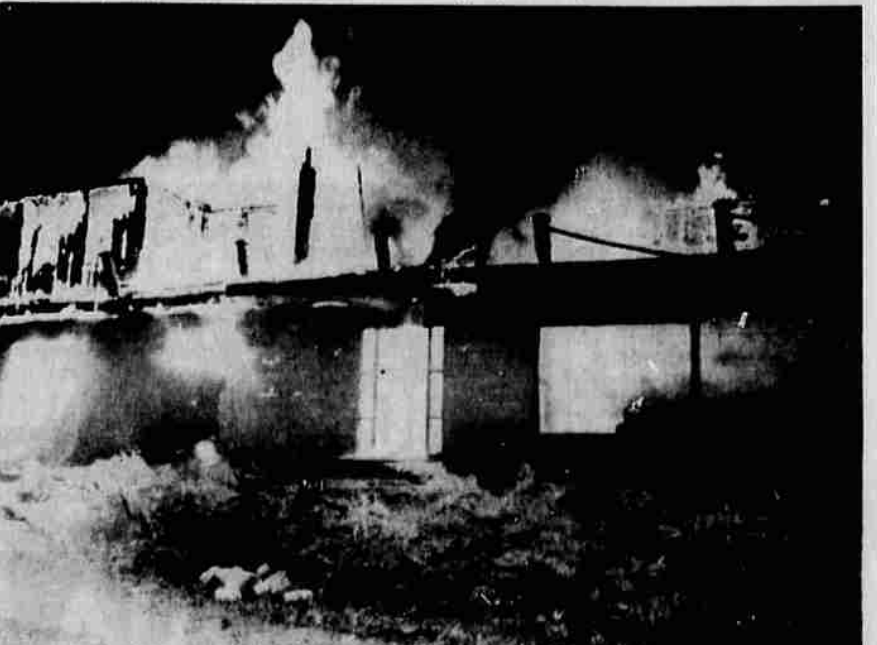
FIRE DESTROYED this 16-room home in North Roseburg early today. The fire was reported about 12:30 a.m. and the house was more than 75 per cent enveloped in flames by the time the fire department arrived on the scene moments later. Although the entire building and all the contents were destroyed, all four members of the Ralph Steel family were away from home when the fire broke out and there were no injuries. (News-Review Photo By Bill Sparks)
