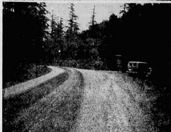
CALCIUM CHLORIDE as a dust retardant on 18 miles of the South Umpqua Road upriver from Tiller has been applied by crews of the South Umpqua Ranger District shown above. Following experimentation with three types of dust retardant in applications last year, part of a dust oil coat applied by a contractor, decision was made to use the dry calcium chloride treatment this year. It is being spread by use of a farm fertilizer spreader attached to a forest service truck. Lower picture shows the appearance of the road after cars have gone over the newly-treated surface. Rainfall of .55 inch on the second day of the project, caused suspension of the application that day, but was beneficial, said Ranger Hillard M. Lilligren, as it permitted grading and shaping up of the road without use of a water wagon. (Forest Service photos)
