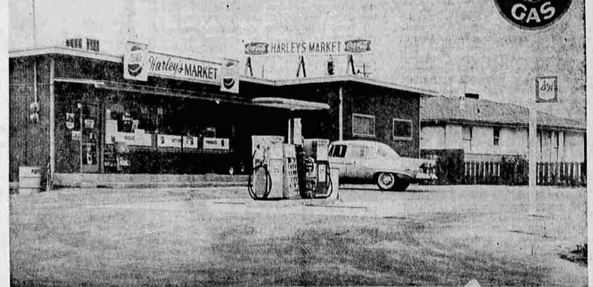
OPEN HOUSE is being held today for Harley's Market in Winston, which has just added service station facilities to its business. The open house will continue until 8:30 p.m. tonight. Gasoline pumps and blacktopping of the parking
