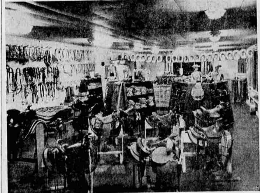
ALLEN'S WESTERN GOODS has moved from Winston to Roseburg and is located in the former Munnell & Sherrill Inc. building across Highway 99 from the Southgate Shopping Center. The building offers Willis Allen and his wife, Frances, much larger space for display of their western supplies, and also provides space as a workshop on leather goods and items for the horse.
